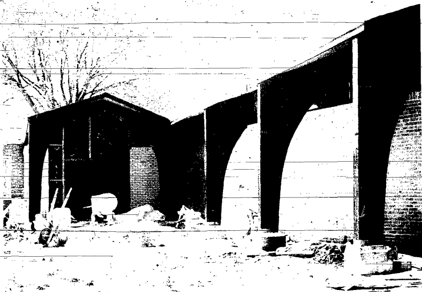
Ladders and wheelbarrows will soon be replaced by worshippers as the Laurel United Methodist Church nears its completion date of June 18.
